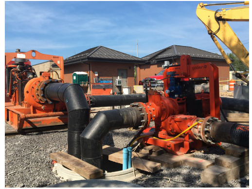
The temporary bypass system, which included a Godwin Dri-Prime CD300M 12-inch diesel pump and Godwin Dri-Prime CD225M 8-inch electric pump, operated continuously for three months during equipment upgrades at the John Street lift station (seen in the background).
