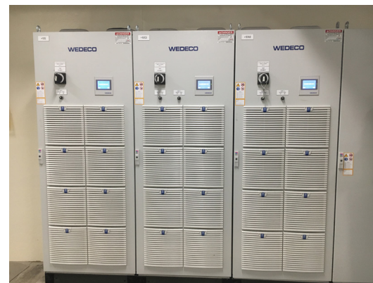
Cabinets house the ballasts to protect important electronics, which are out of the water channel, while also enabling quick access for maintenance.
