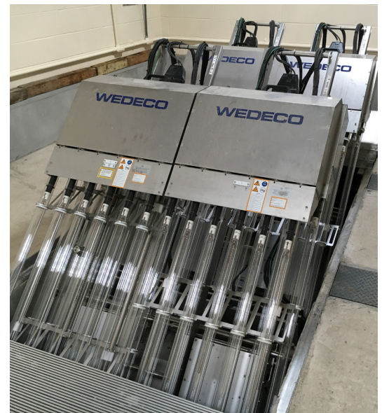
The Duron UV system's natural incline and automated lifting mechanism provides the most ergonomically-friendly maintenance on the market.
