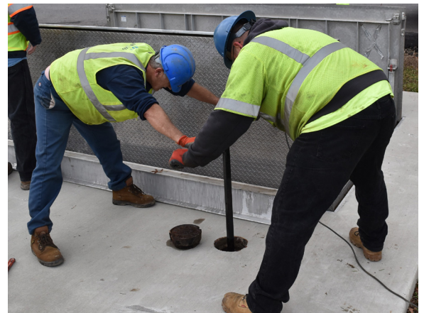
Valve condition assessment
