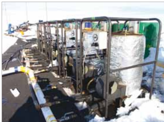
183 barrels of jet fuel and 5 barrels of gasoline were needed to drill the access holes.
