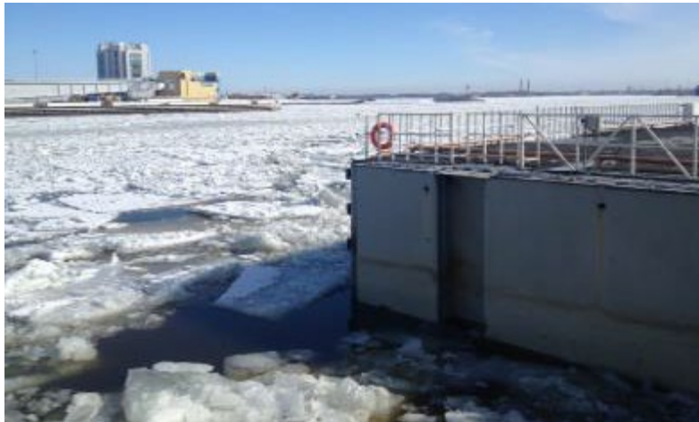
Barrier and Dam operations
