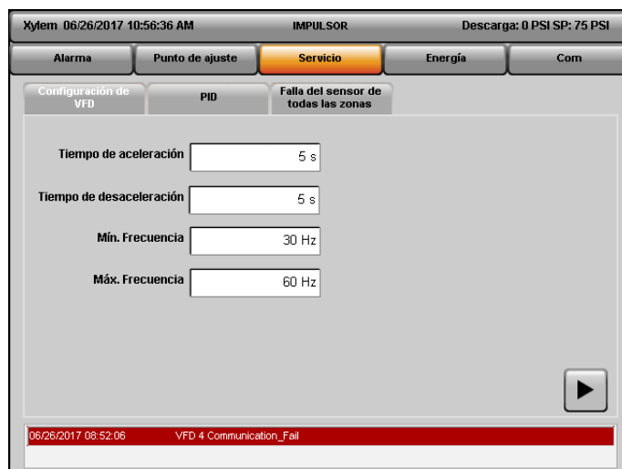
Figura 5.5.11: Control de VFD
