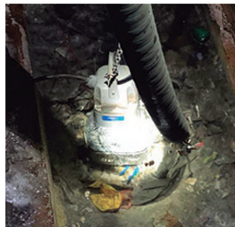
Pump installed and running.
