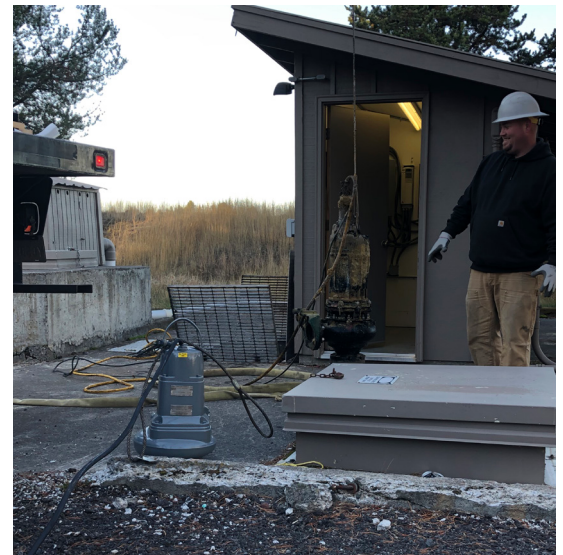
Contractors prepare to install a Concertor pump at Lift Station 3.
