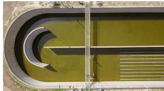
An existing oxidation ditch was retrofitted with a new Sanitaire Bioloop treatment solution, including Flygt adaptive mixers.
