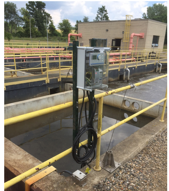
Tank side controls provide easy access to a host of mixer functions.
