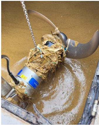
Intelligent mixer senses debris and slows down to dislodge from the propeller.
