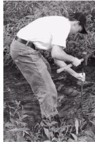
Securely insert a piece of mounting material into the center of the channel.
