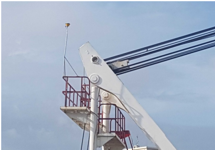
FIGURE 2. GPS Antennas Installation
