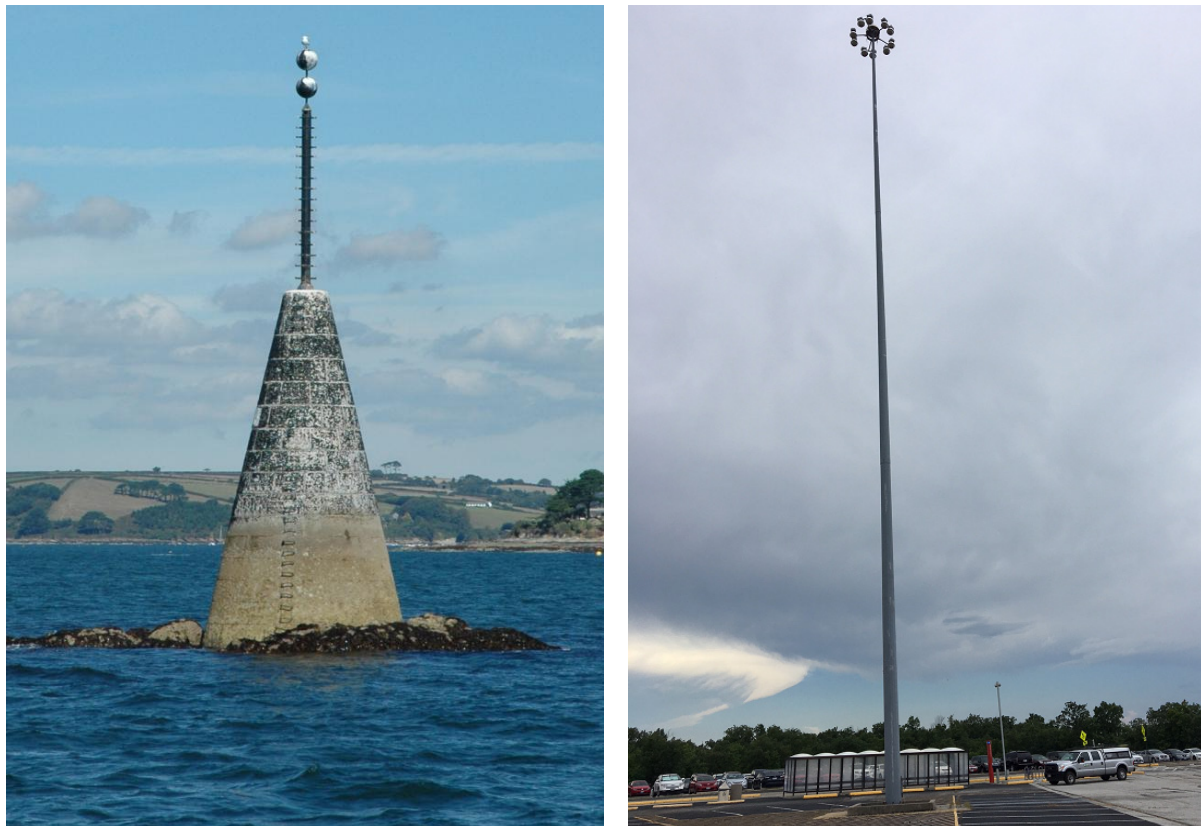
FIGURE 3. Daymarks and Light Poles Make Good LIDAR Patch Test Features.
