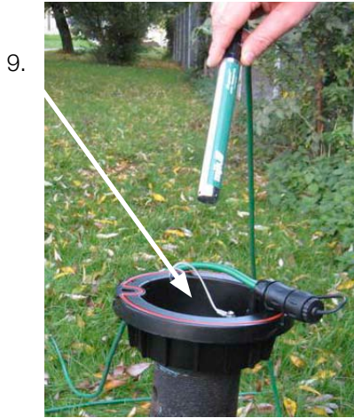
Figure 9. Immerse the Pressure Transmitter
