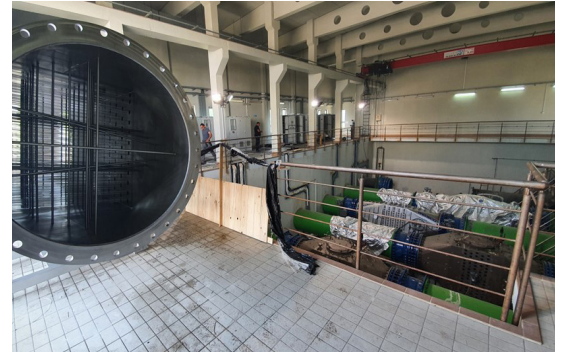
Insertion of the new Wedeco K143 reactors.
