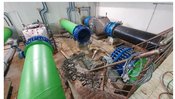
Removal of old units.
