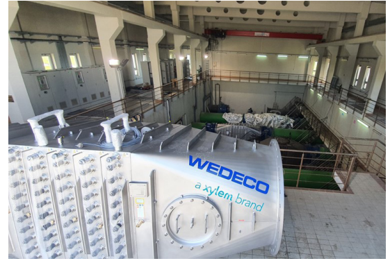
Insertion of the new Wedeco K143 reactors.
