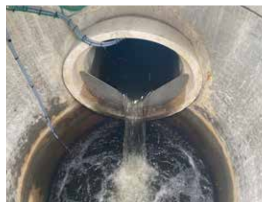
Figure 8 Stormwater Event Operation
