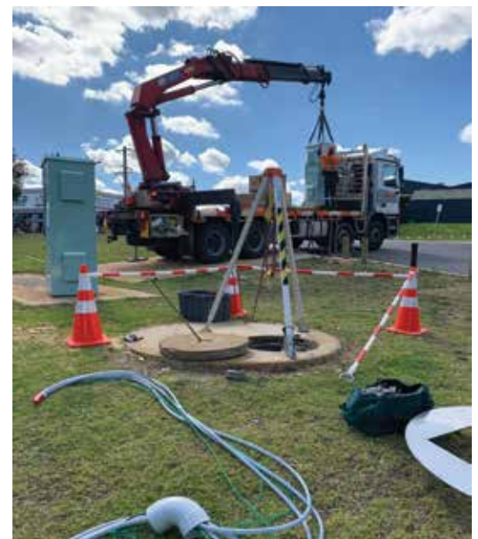
Figure 2 Monitoring Station Construction
