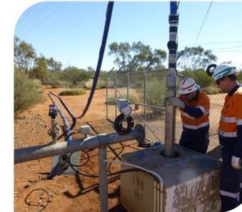
Lowara borehole pump installation
