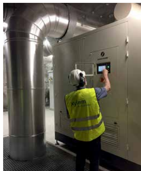
Xylem employee assisting in startup of MAX600 (400kW) blower.
