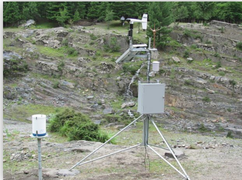
ENVIRONMENTAL MONITORING STATION
