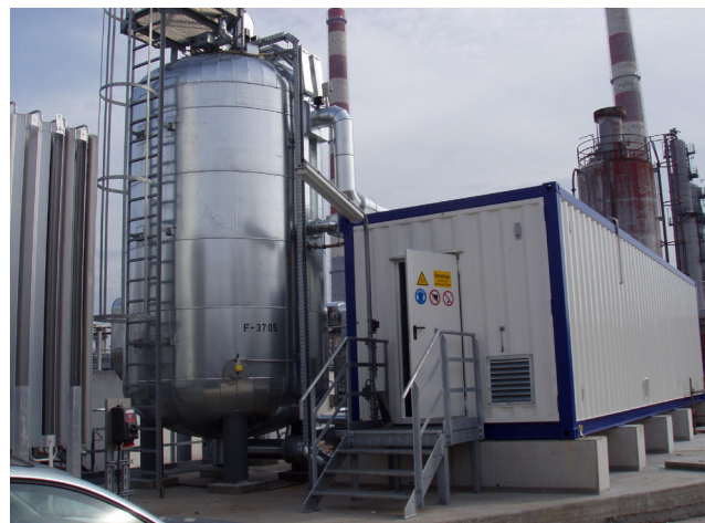
Container installation and reaction tank
