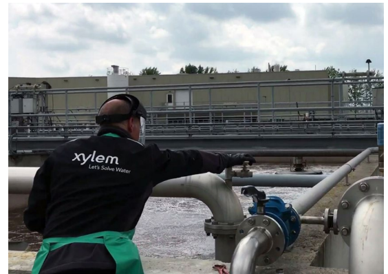
Service engineer prepares for Diffuser Liquid Cleaning
