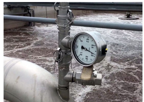
Immediate result with 40 mBar back pressure reduction on the blowers
