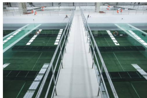
Leopold Type S Underdrain gravity media filtration system
