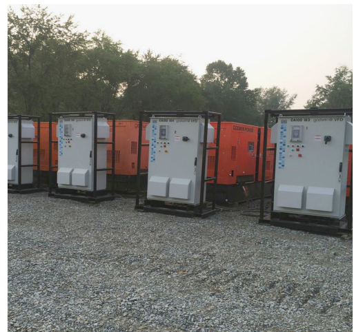
As part of the rental solution, Godwin VFDs and Generators - one set for each of the five Flygt pumps - were integral to the bypass operation.
