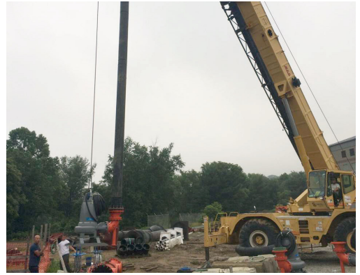
Once the piping was affixed to the Flygt pump, it was lowered into the wet well.
