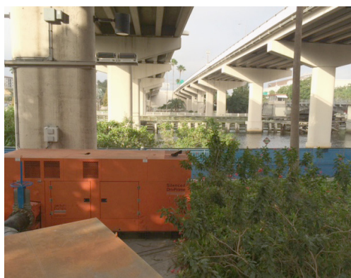
Space was limited under the expressway and along the river.
