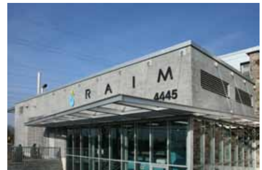
RAIM (La Régie d'aqueduc intermunicipale des moulins) treats and distributes high quality potable water to its users in the cities of Terrebonne and Mascouche.
