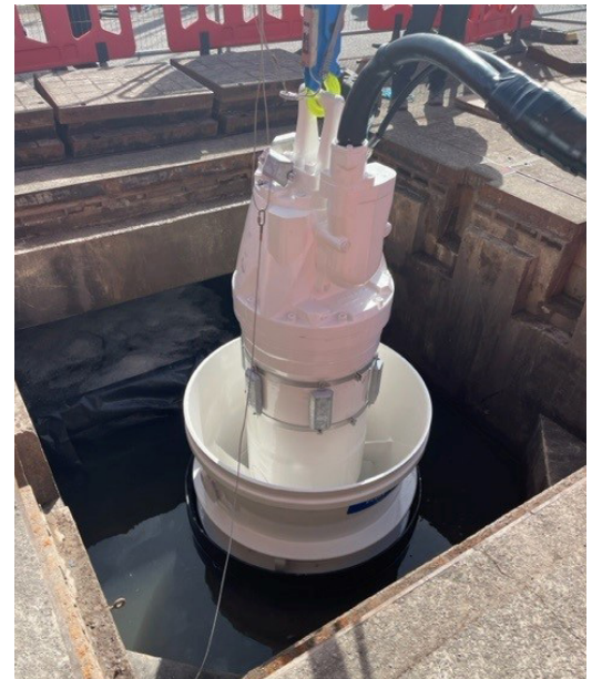
Figure 4. Pump installation.
