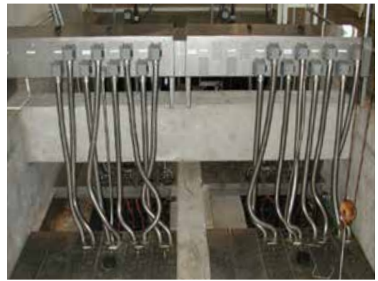
Wedeco UV system divides UV lamps between two channels
