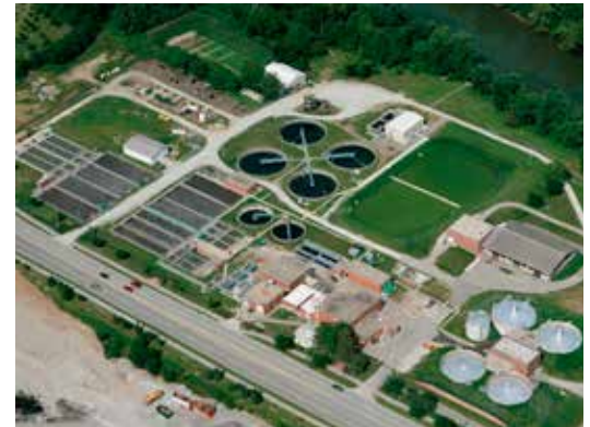
Aerial view of Carmel WWTP
