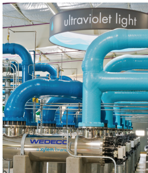
Xylem’s Wedeco LBX 1000 UV Disinfection System at Silicon Valley AWPC
