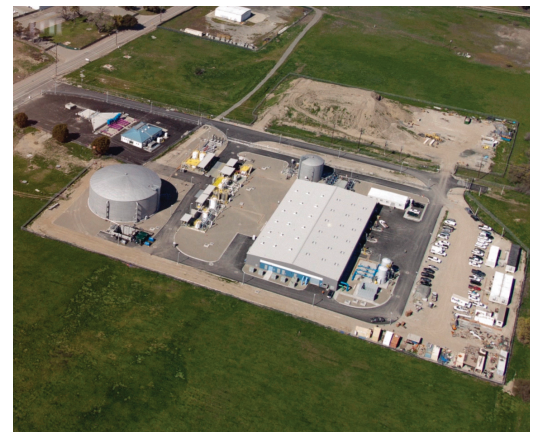
Silicon Valley Advanced Water Purification Center
