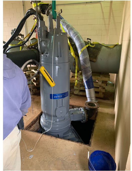
The Flygt 3231 submersible pump is lowered into the pump wet well.
