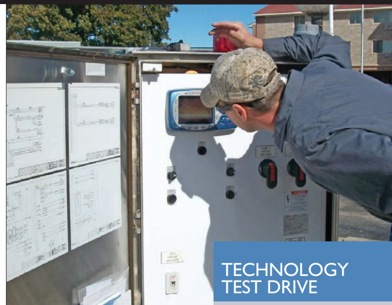
Travis Walker of the City of Beaver Dam shows the operation of the MultiSmart unit that operates a lift station. (Photography by Matt Gunn)
