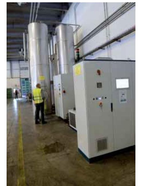
HSE and Xylem technicians worked in close contact to identify the best solutions
