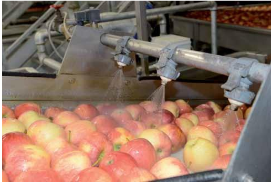
The effectiveness and efficiency of ozone treatment have been verified in the field after 6,000 hours of operation
